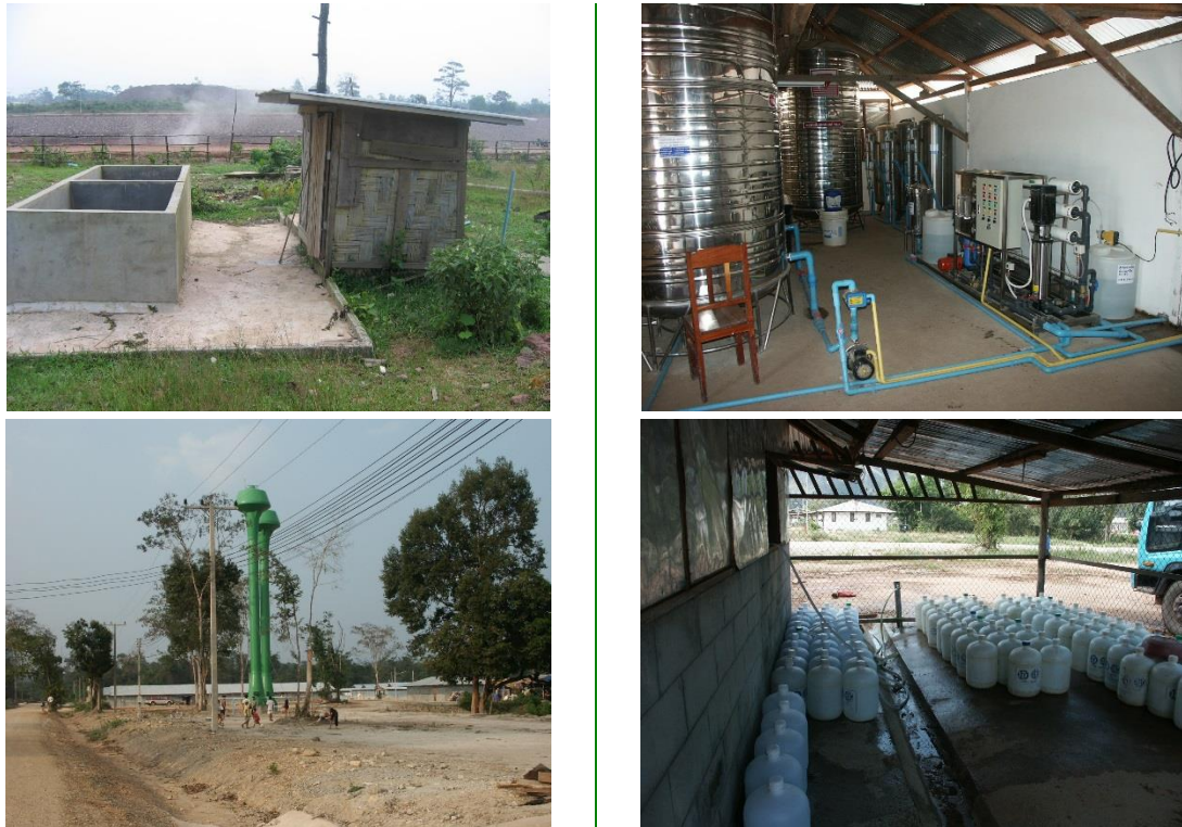
Figure 6: (a) Top left-hand picture: toilet (right) and water container for washing and personal hygiene purposes (right); (b) Top right-hand picture: drinking water treatment plant in the main camp; (c) Bottom left-hand picture: water tower in the main work camp – as a direct drinking water source for the main camp and an indirect one for secondary camps (to which drinking water is transported via trucks and water tanks, see picture d); (d) Bottom right-hand picture: water tanks for transporting drinking water from the main camp to secondary work camps.
