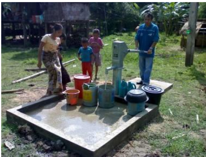
Figure 7: one of the 500 boreholes equipped with Afridev pump
